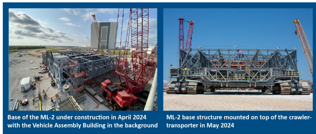
Figure 8: Construction of Mobile Launcher 2 at Kennedy Space Center
