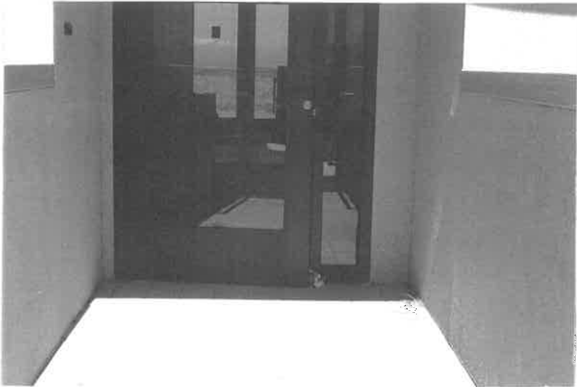
NEWSPAPER IN DOOR AT NAS SUPPORT BUILDING B
