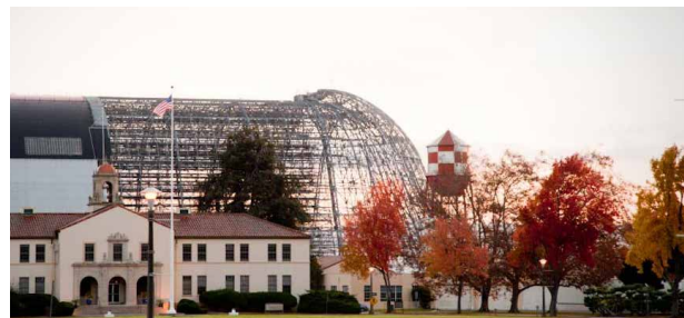
Historical Building 17 at Ames Research Center, with the Hangar One deskinning project visible in the background
