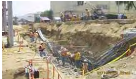
2008 duct bank collapse at JPL during which subcontractor employees were placed at risk during repair work. Trench cave-in not reported to the JPL Occupational Safety Office for 3 days.
