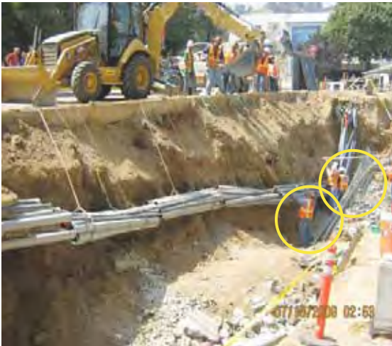
2008 duct bank collapse at JPL during which subcontractor employees were placed at risk during repair work. Trench cave-in not reported to the JPL Occupational Safety Office for 3 days.
