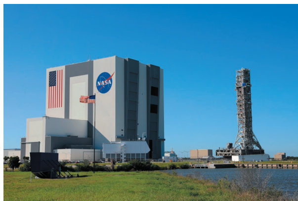
The mobile launcher for the Artemis I mission, atop crawler-transporter 2, arrives at the Vehicle Assembly Building at NASA's Kennedy Space Center in Florida on October 30, 2020.
