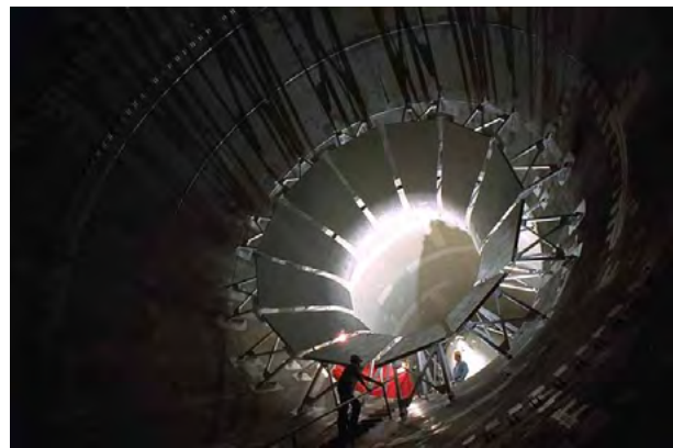
Work being done on the diffuser and contraction vanes in the Unitary Plan Wind Tunnel at Ames Research Center
