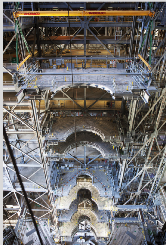
Vehicle Assembly Building for the SLS, Kennedy Space Center
