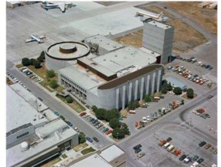
Except for the Vertical Motion Simulator, which is still active, building N243 has been refurbished into primarily office and lab space.
