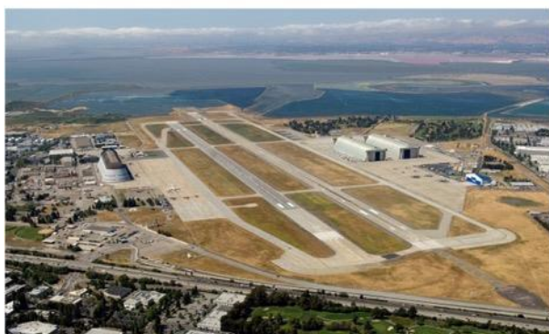
Aerial view of Moffett Field. On the left is Hangar 1 prior to removal of hazardous covering.
