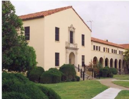
Building 19 has been refurbished into the NASA Exchange Lodge and a multi-tenant office building.
