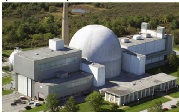
Space Power Facility
