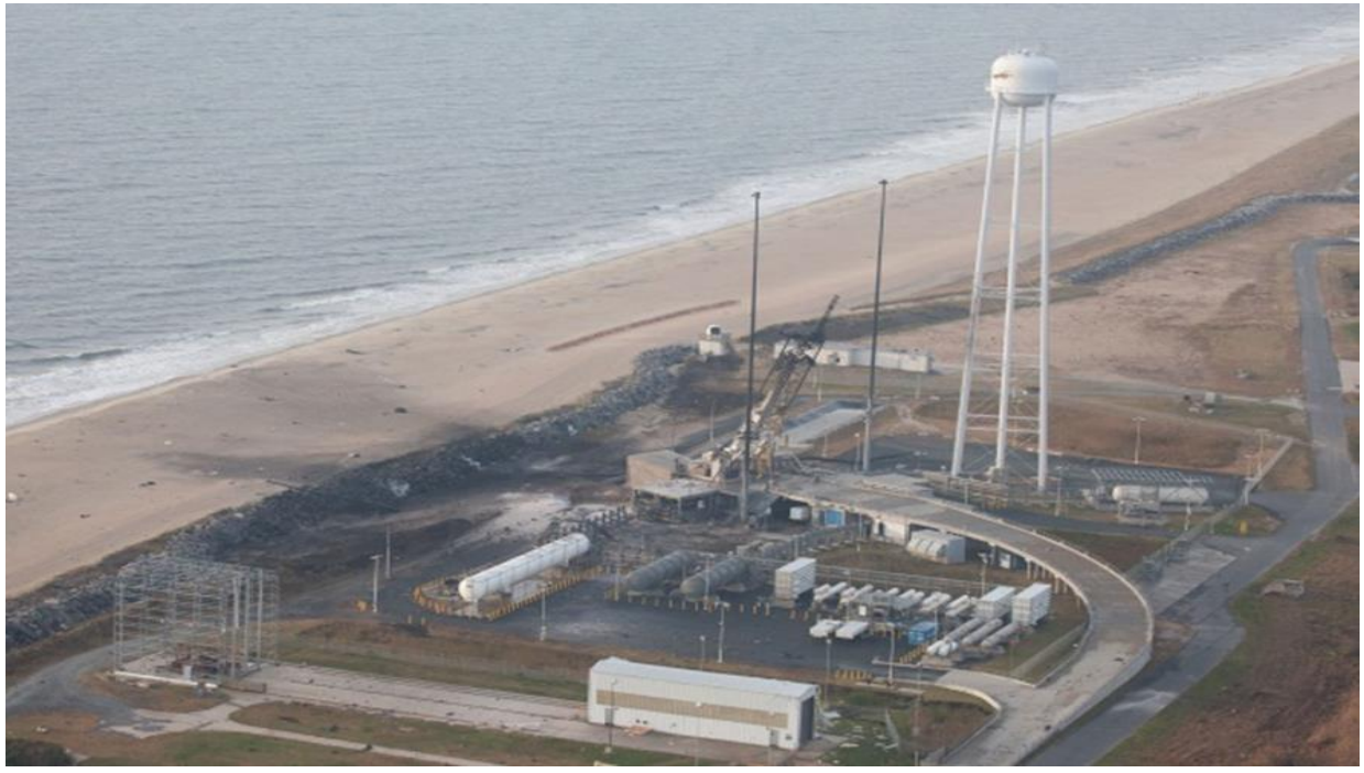
Figure 2: Damage to VCSFA Launch Complex at Wallops
