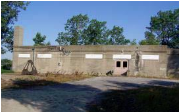
Rye Beach Pump Station
