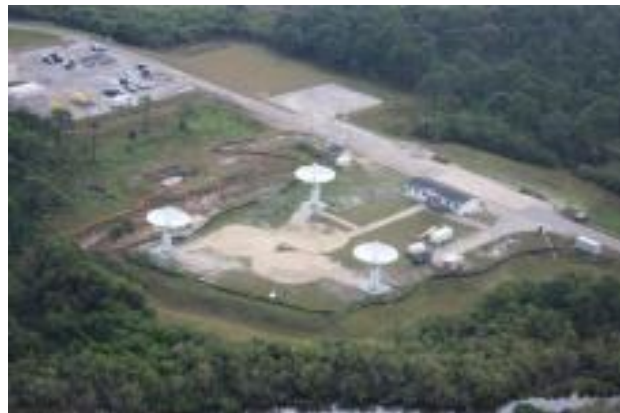
Figure 9. KaBOOM Radar Array
