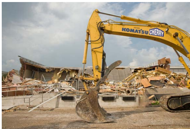
Figure 4. Demolition of Johnson's Building T-585 July 2012
