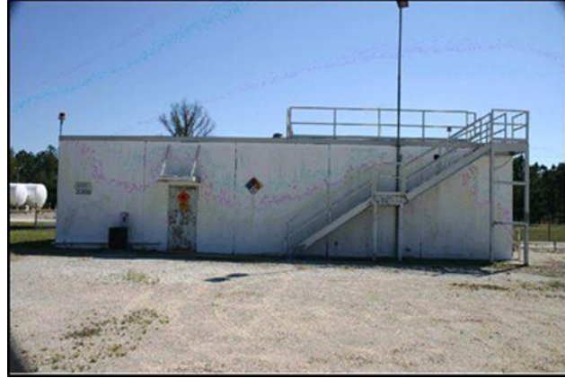
Figure 5. Explosives storage facility building
