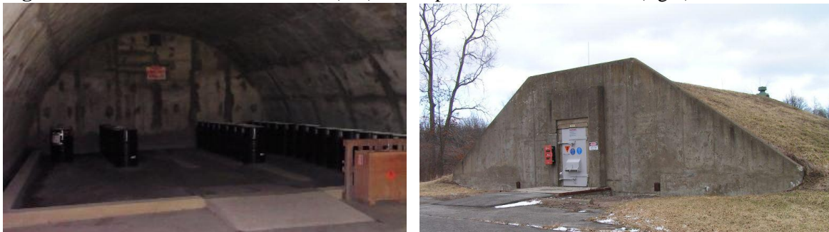
Figure 3. Hazardous chemical bunker (left) and explosive material bunker (right)
