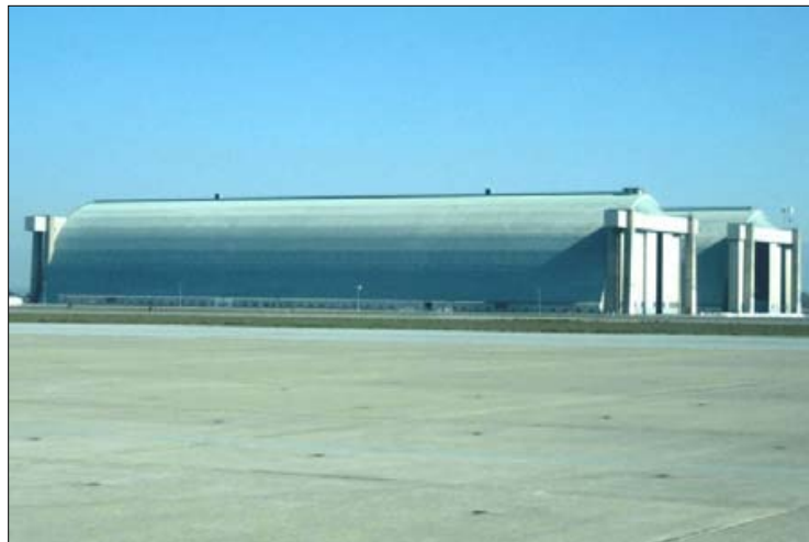
Figure 4. Hangar Two and Hangar Three
